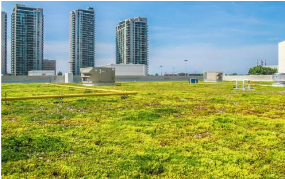
Figure 2. Extensive green roof on Sherway Garden Shopping Centre. Greenroofs.com, 2014.
