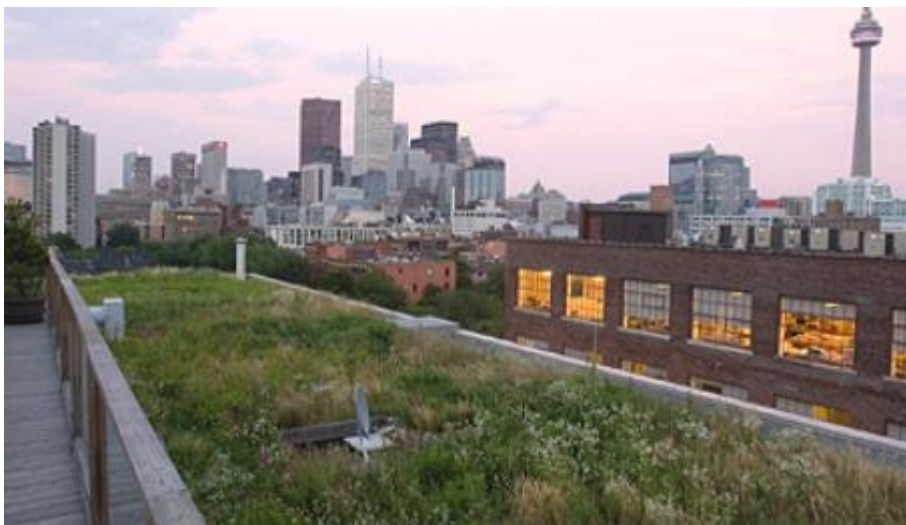
Figure 5. Semi-intensive green roofs of Robertson Building. Less Mess, 2013.
